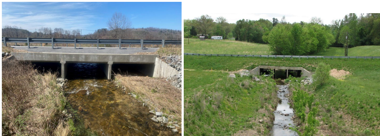
Figures 4 and 5. Benching into box culvert (left, Transylvania County, #870012, Hogsed Creek) and benching with bank sloping (right, Mecklenburg, I-485 vicinity, unnamed tributary).
