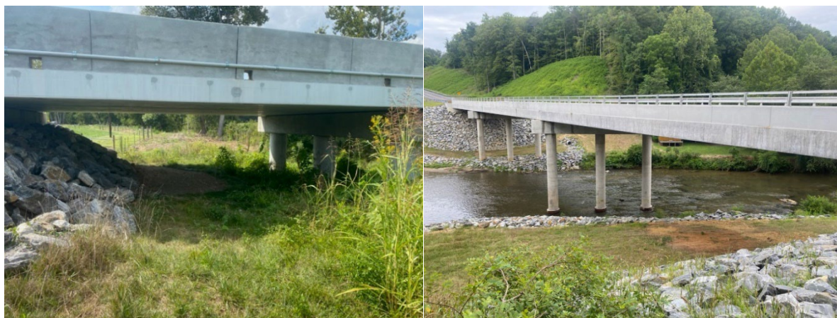
Figures 7 and 8. Unarmored floodplains under bridge in Iredell County (left, #480212, Patterson Creek) and large bridge in Stokes County (right, #840008, Dan River).
