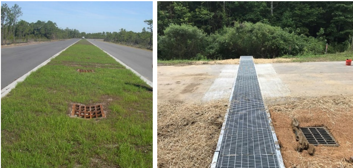
Figures 20 and 21. Grate in median of wildlife culvert, EF Middleton Blvd Brunswick County (left) and open grate crossing Ashe County.
