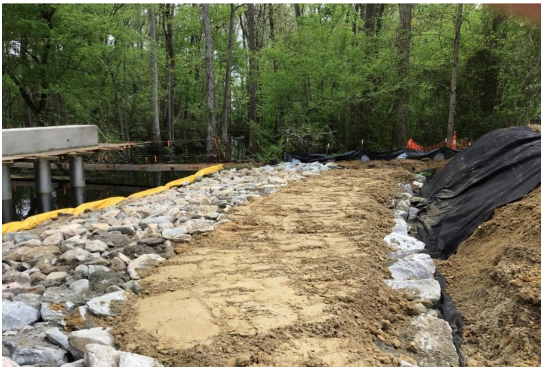
Figure 13. Construction of bench over embedded rip rap (Edgecombe County, # 320113, Otter Creek).
